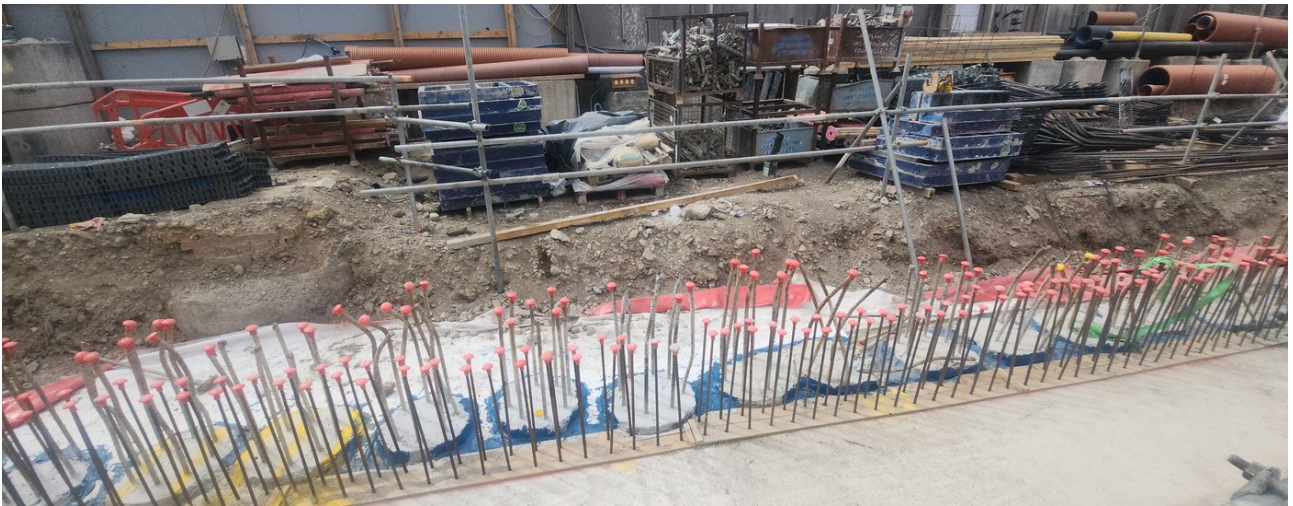
Concrete operations running alongside structural works on a live multi phase site.
