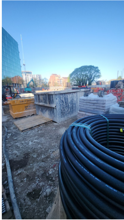
Grouting and borehole completion works, part of the sequence that has to be documented and signed off.
