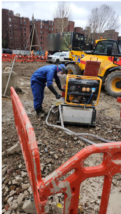
Close quarters drilling access. Confined yard working is one of the most common access risks on retrofit drilling.
