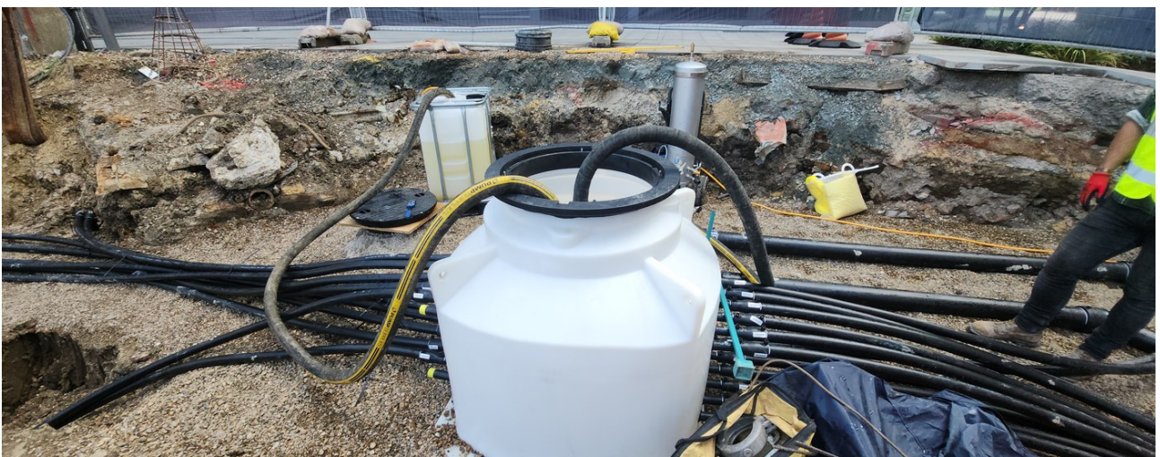
Site management during an active drilling phase, groundworks and drilling plant sharing the same footprint.
