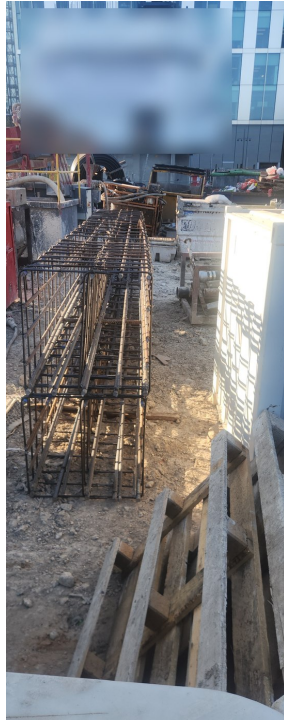
Reinforcement and groundworks ahead of a drilling and piling sequence on a larger scheme.
