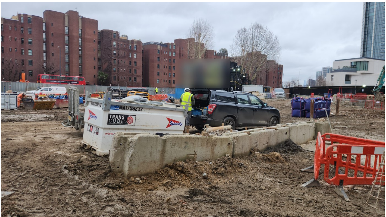
Drilling in progress. Sequencing a rig safely around an occupied site is a RAMS and phase plan discipline, not an afterthought.
