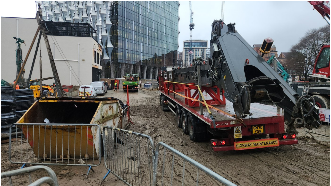
Rig set up and casing ready for a ground source borehole, social housing retrofit programme.
